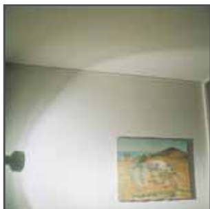
Incorrectly positioned spotlights
